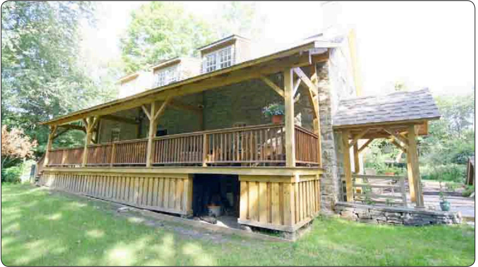
WOGAN'S WORK ON THE CLASSIC STONE DUTCH COLONIAL IN STONE RIDGE, WHERE HE LIVES WITH HIS FAMILY, INCLUDED THE ADDITION OF A PORCH THAT CAN BE REMOVED AT ANY TIME WITHOUT DAMAGE TO THE HOUSE.
