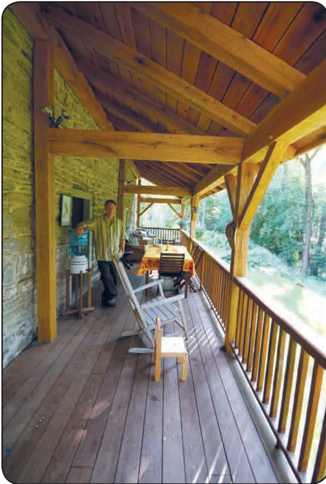
WOGAN DIDN'T WANT TO BOLT THE PORCH INTO THE STONE TO RETAIN THE HOUSE'S INTEGRITY SO HE BURIED CONCRETE FOOTINGS ON WHICH TO MOUNT THE STRUCTURE, BOLTING THE PORCH AT THE EAVES ONLY.
